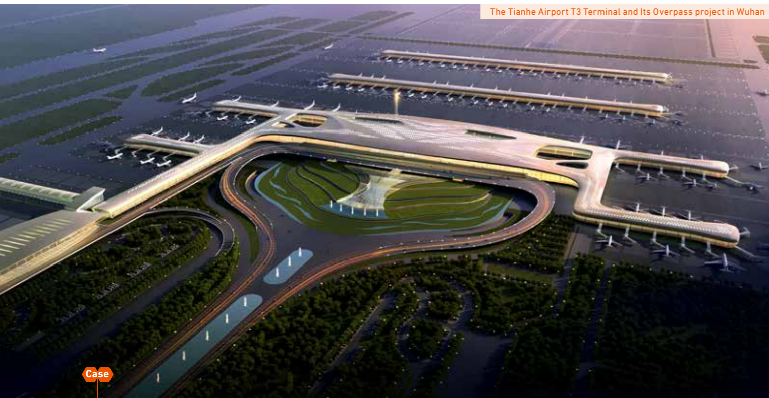
The Tianhe Airport T3 Terminal and Its Overpass project in Wuhan
